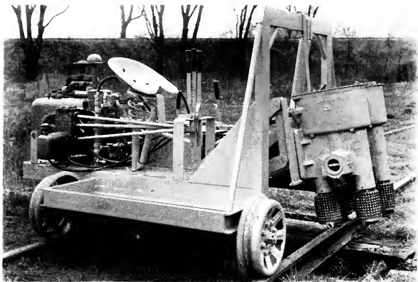
Tie renewal machine.
